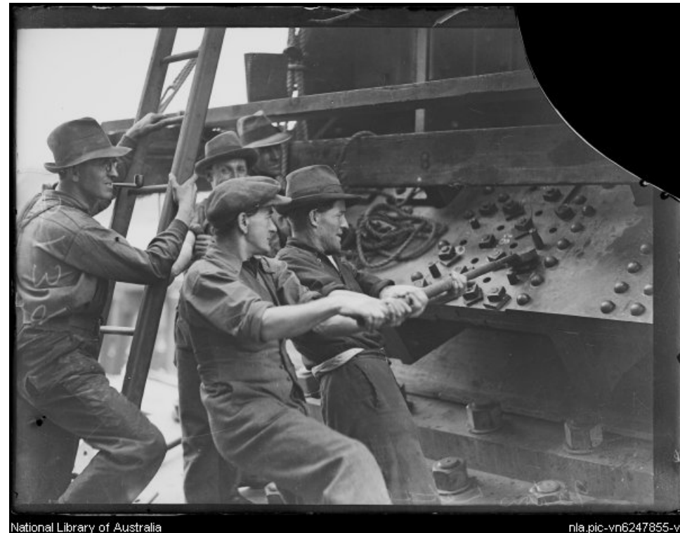
Construction workers tightening the bolts on the Sydney Harbour Bridge, ca. 1931
